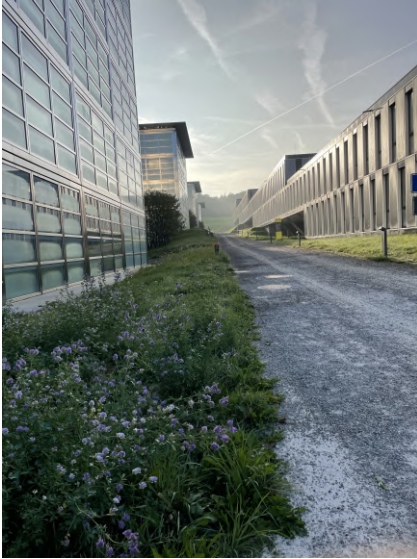
Figure 4.6: HCI building (on the left), the most expensive non-military building in Switzerland at the time of its completion in 2004. [12]
